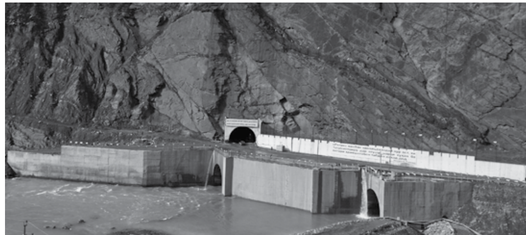
A general view of the Rogun hydro-electric dam, about 100 km northeast of the Tajik capital Dushanbe,
